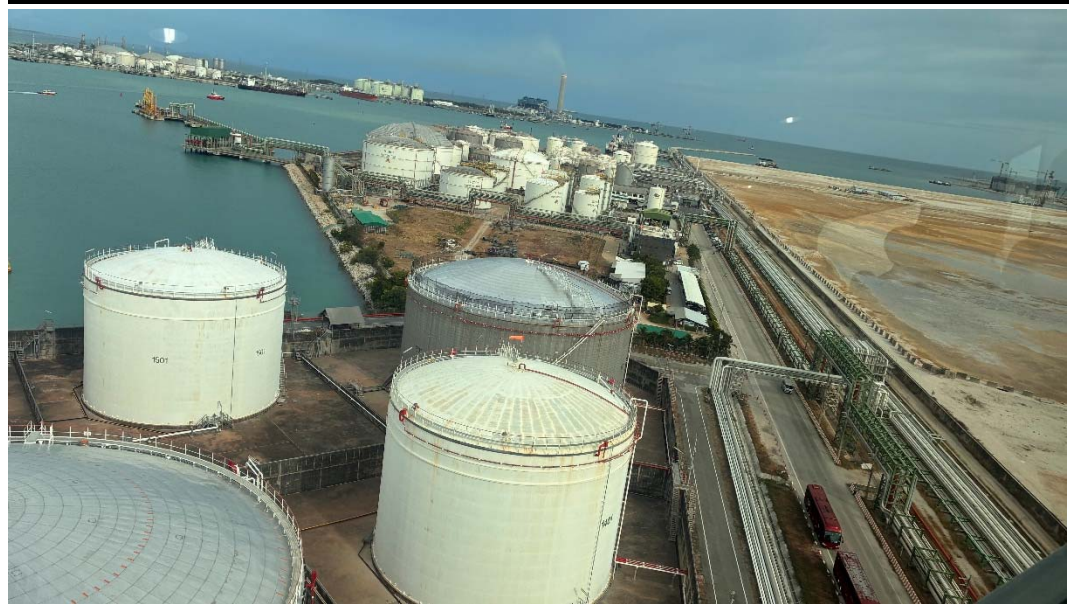
Figure 3: PTT Tank Terminal
